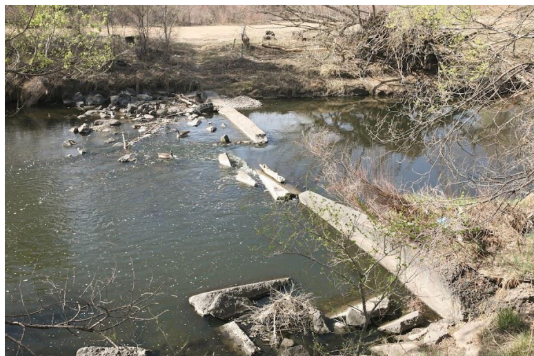
Failed concrete weir on Clear Creek
